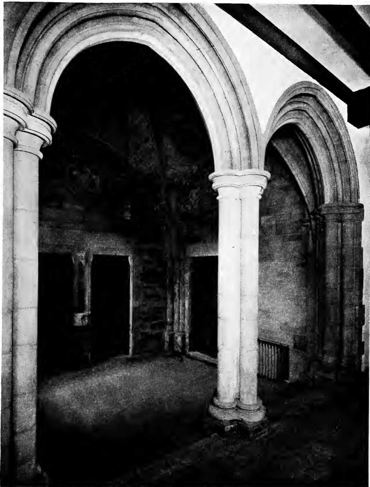
SYNOD HOUSE, CATHEDRAL OF ST. JOHN THE DIVINE, NEW YORK MESSRS. CRAM, GOODHUE & FERGUSON (BOSTON OFFICE), ARCHITECTS
